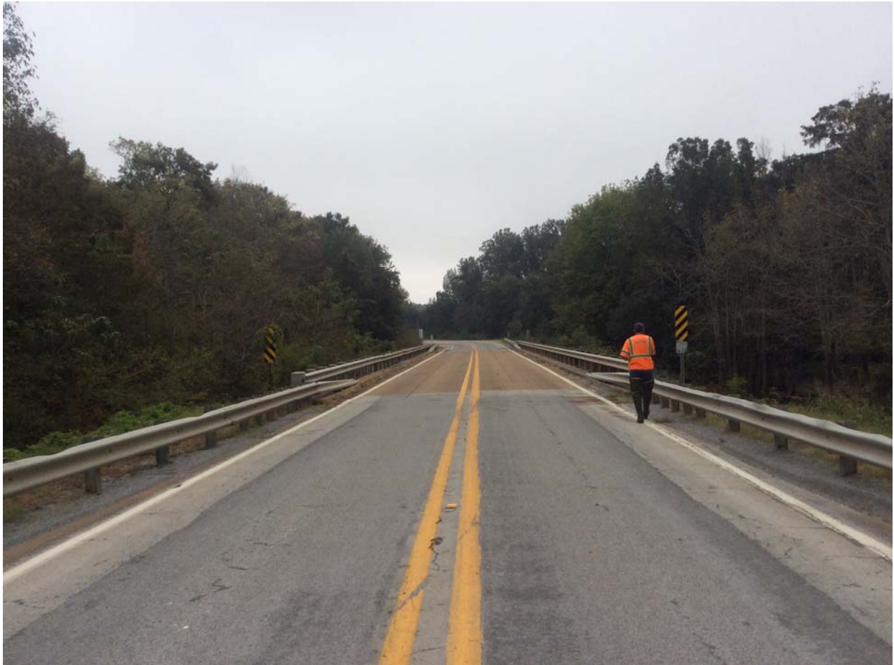
Note: 4" ACHM overlay on bridge deck.
